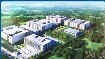
Beijing-Tianjin-Hebei Data Centers
