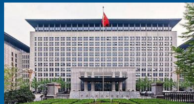
National Ministry of Commerce Data Center
