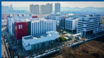
Data Center Cluster in Shandong Province
